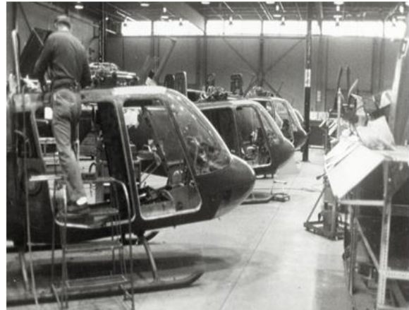
Title: Repair facility of Bell Huey Helicopter Fig No 6
